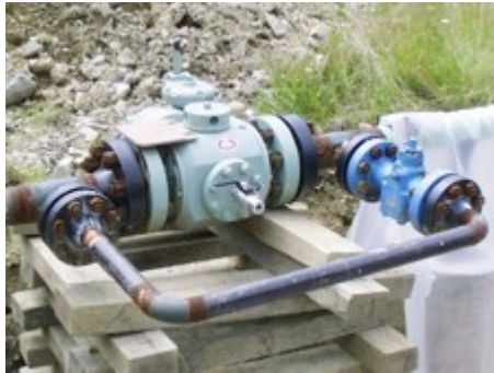
Argus 6" Pig Launching Valve being installed with bypass loop.
